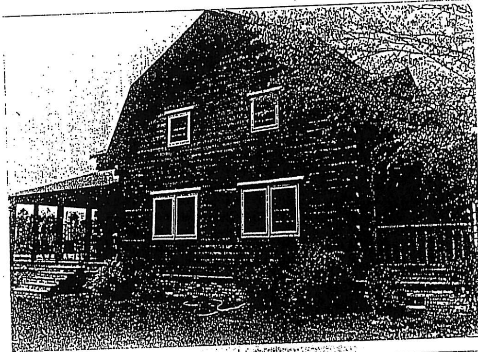
UPPER PHOTO: View of the gabled end of the house showing the configuration of the logs and gambrel roof. The majority of the leaks are coming in through the gabled end walls.
