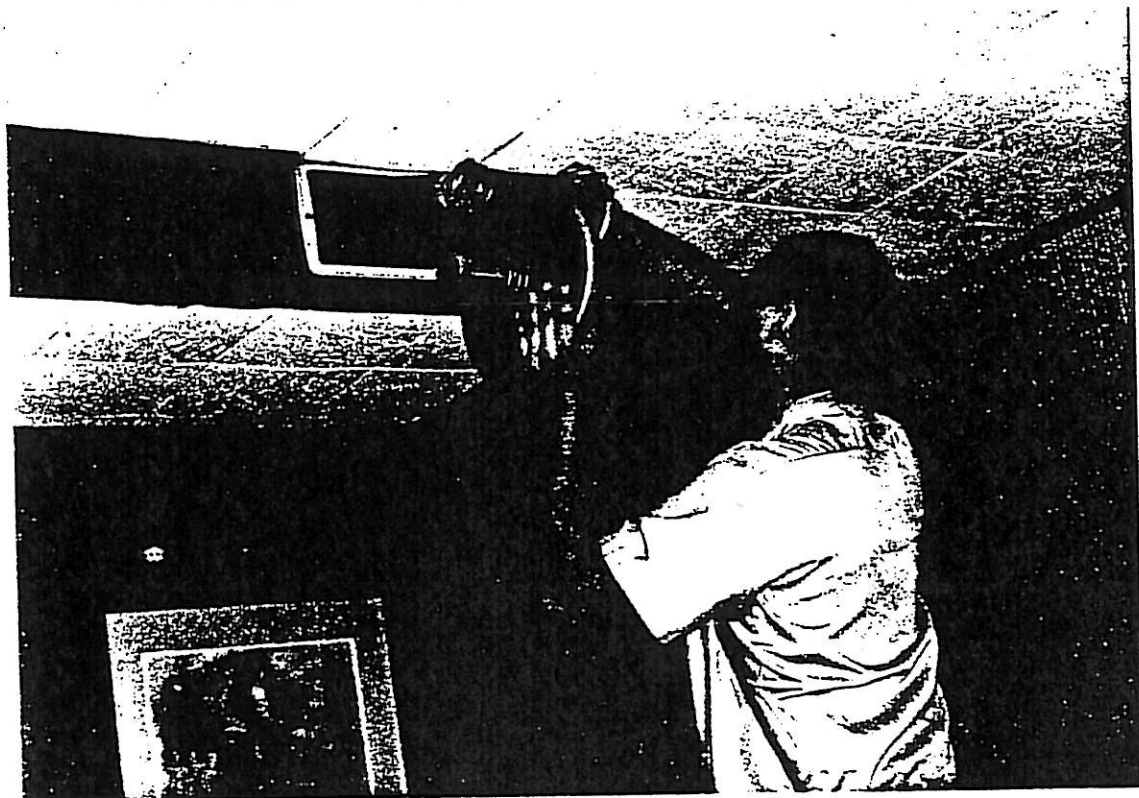
Technician "blowing down" soffit register
