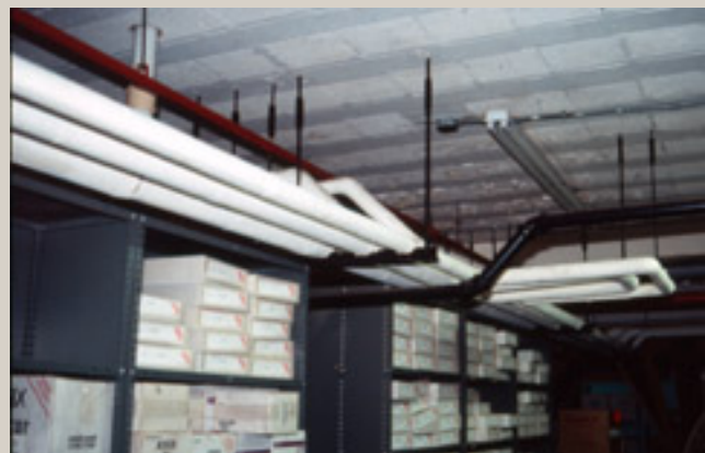
Overhead pipes with asbestos insulation
