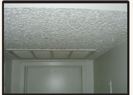
Textured plaster ceiling with asbestos
