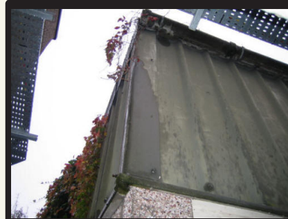
Damaged asbestos cement siding
