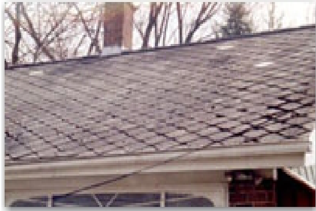
Asbestos roofing materials
