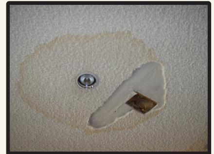
Asbestos in textured ceiling
